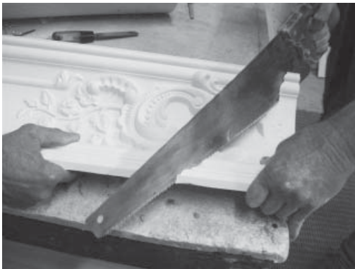
Step 3. & 4. Using either a compound miter box or hand saw, cut each piece at 45 degree angle using the molded tab as a guide.
